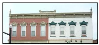
Original windows and opening should be maintained, if replacement windows are installed they should properly fit within the original opening
