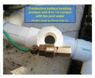
INSTALLS BELOW WATER LINE MINIMUM 9 SQ INCHES OF SURFACE AREA UL LISTED
