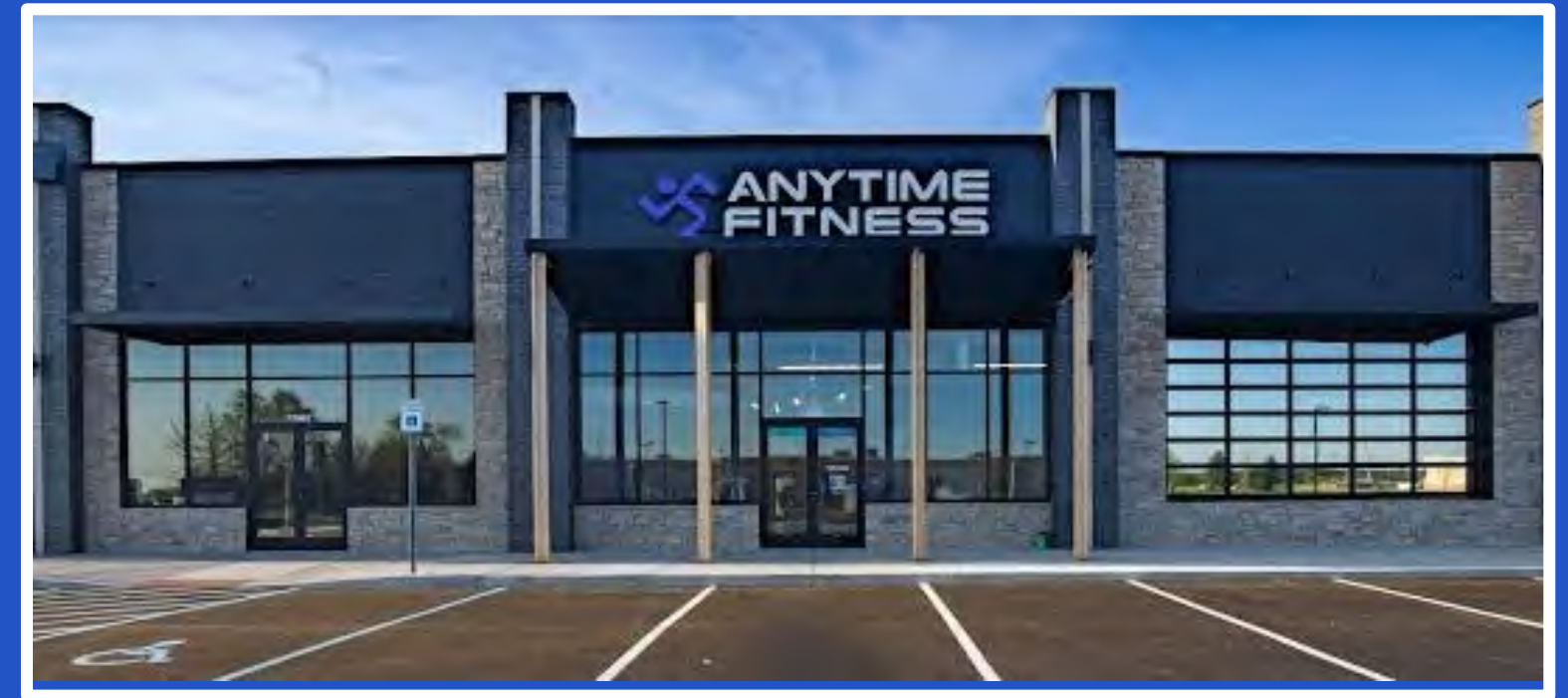
Anytime Fitness New Construction
